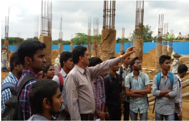
Construction site, Kuvempu Trust Road Gokulam ,Mysore
